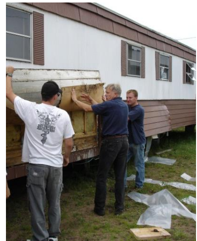
Loosening siding for wall insulation: Remove screws at the bottom of the metal siding. Before installing insulation, fasten the siding sheets together at the bottom with a short sheet-metal screw.
