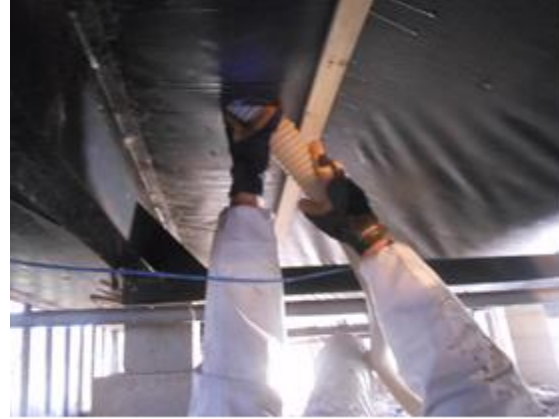
Blowing insulation from under the home: A large diameter fill tube fills cavities rapidly from underneath.
