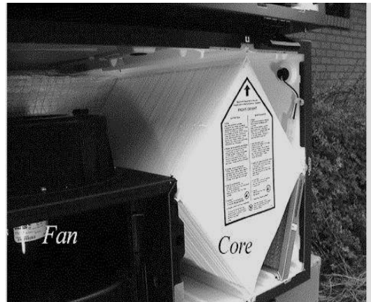
Polyethylene HRV core: This flat-plate counter flow heat exchanger slides out for cleaning.
