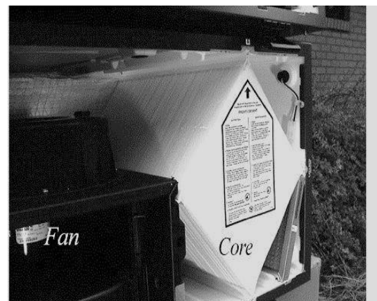
Polyethylene HRV core: This flat-plate counter flow heat exchanger slides out for cleaning.
