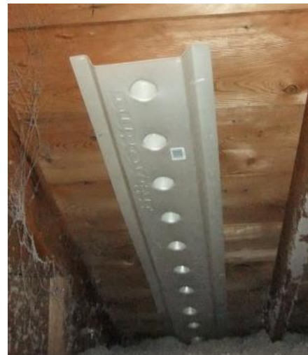
Soffit chute: Allows installation of maximum amount of insulation in this cold area. Also prevents wind washing and airway blockage by blown insulation.
